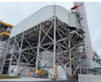
▲ The wet dust collector of CR Power Wenzhou Power Plant
